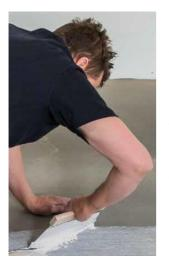
For the installation of Xtrafloor® Flex Pro: lay the sheets butted, edge-to-edge, at a 90 angle to the laying direction of the new floorcovering.
